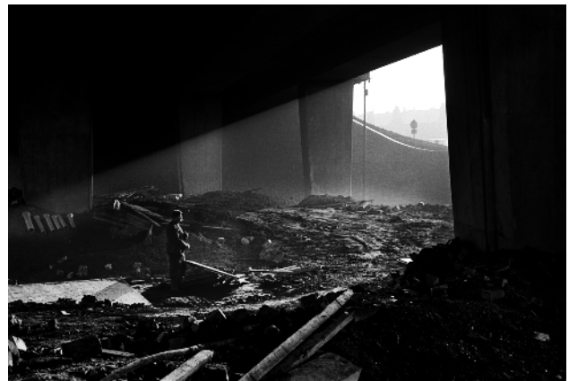
Townhead Interchange during Construction (1968)
